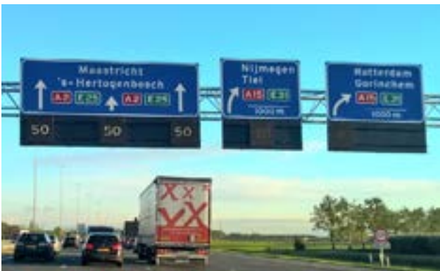
Image 7: Dynamic speed limit per lane, and static speed limit per time period: 50, 70, 100, 120 or 130 km/h.
