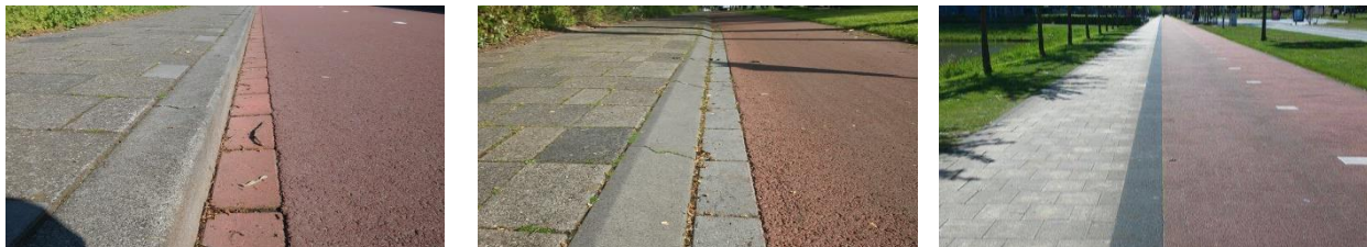
Figure 1. Kerb types applied in the Netherlands (From left to right: right angled kerbs, sloped kerbs, levelled kerbs)
